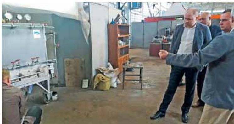
Test launch of synthetic gas facility
